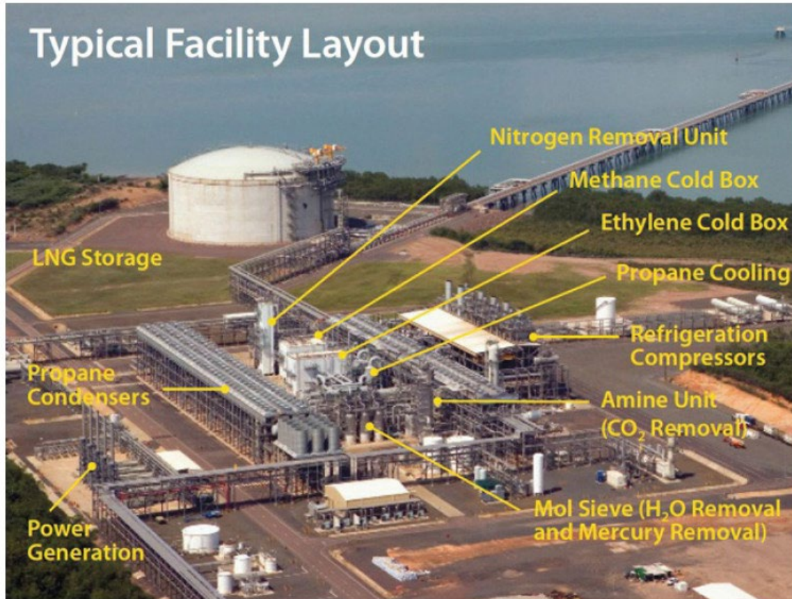
Key components of the Optimized Cascade process in use at Darwin LNG
