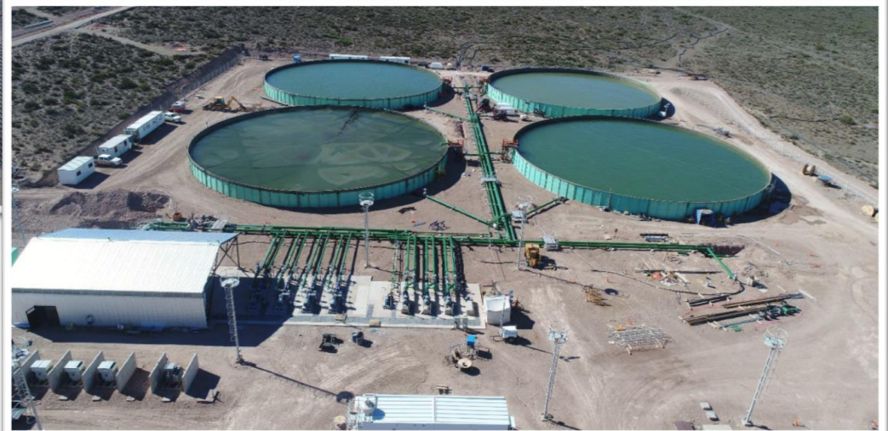
Water Storage & Transfer 20,000 m 3 capacity
